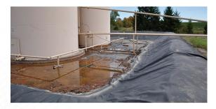
Our geomembranes are specially formulated to remain highly flexible and resistant to cracking or puncture on rough or uneven surfaces — even across the entire range of normal operating temperatures. They can also be formulated to be highly resistant to degradation from ultraviolet light, making them suitable for a wide range of applications that are exposed to the elements.
