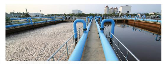
Wastewater containment generally includes large, shallow basins for settlement, treatment and storage. These basins must not only be watertight, but impervious to both the harsh chemicals used in the treatment process and the active biological agents in wastewater. Plastatech geomembranes are well-suited for both primary and secondary containment in wastewater treatment facilities.
